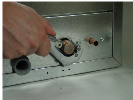
Figure 22. Cut end of connection as shown.
