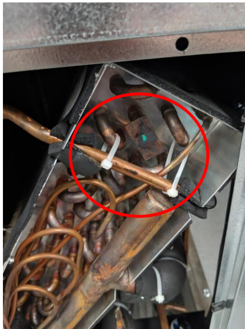
Figure 24. Cut zip ties before installing TXV
