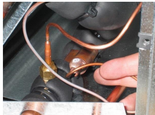
Figure 29. Thermal Measuring Bulb Placed on Copper Tube.
