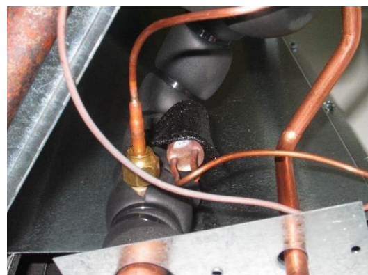
Figure 30. Bulb Secure Clamp and Cork Tape
