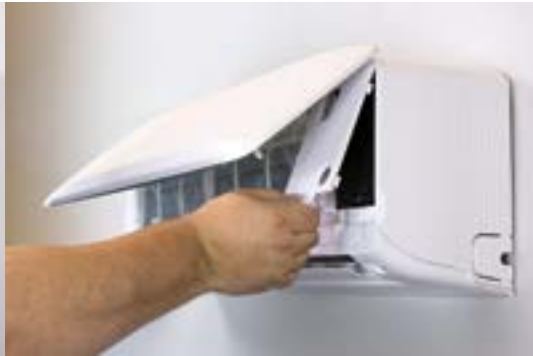
Remove electrical access panels (2)
