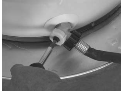
Figure 12 - Draining the old water heater.
