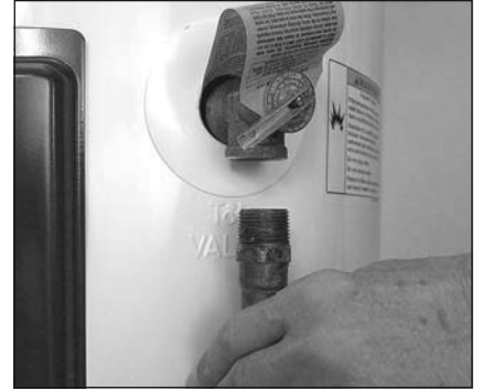
Figure 13 - Removing the T&P Relief Valve discharge pipe.
