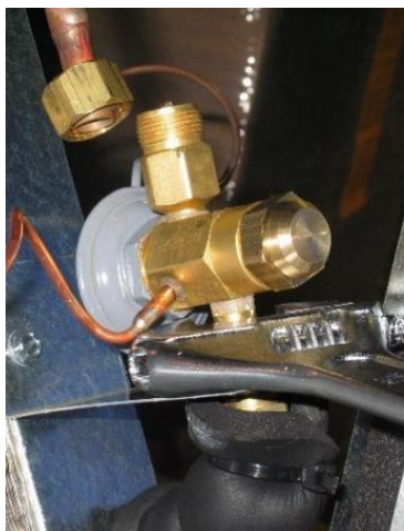
Figure 9. Attaching TXV to Distributor
