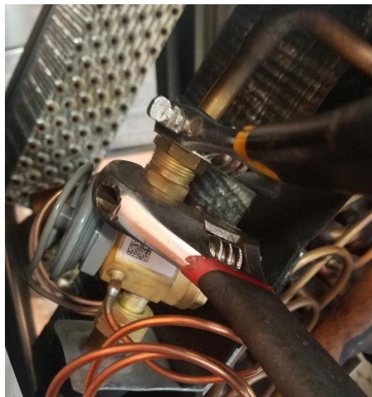
Figure 10. Attaching TXV to Liquid Line
