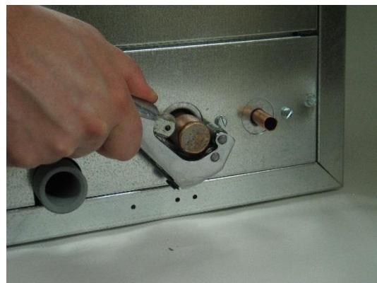
Figure 22. Cut end of connection as shown.
