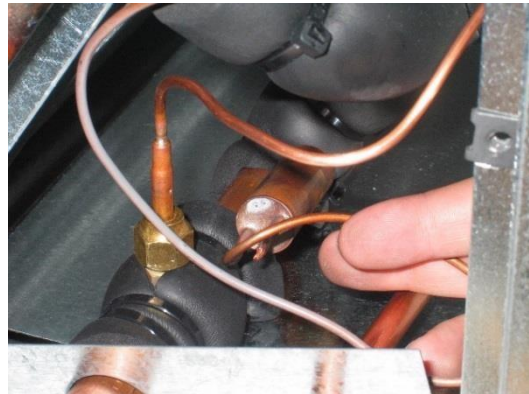
Figure 29. Thermal Measuring Bulb Placed on Copper Tube.
