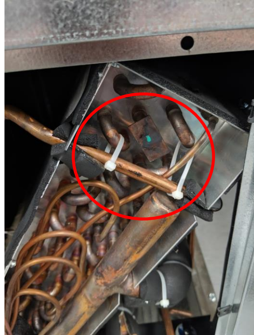
Figure 24. Cut zip ties before installing TXV
