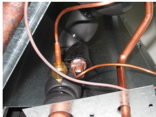
Figure 30. Bulb Secure Clamp and Cork Tape
