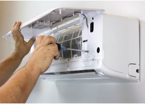
Back out electrical panel screws
