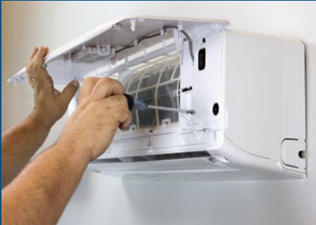
Back out electrical panel screws
