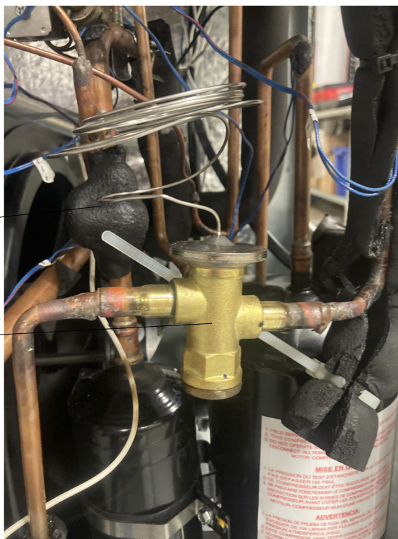
Figure 701 (TXV Valve Replacement)
