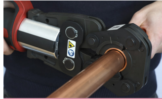
3. Complete the joint with the press tool
