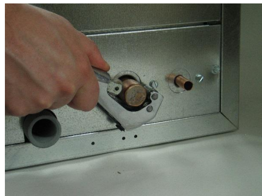
Figure 22. Cut end of connection as shown.
