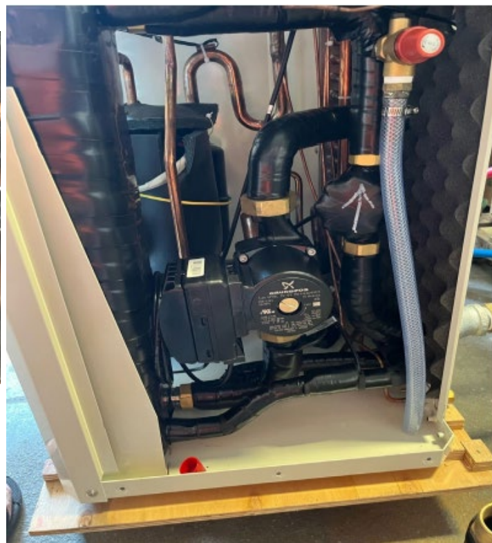
Removing the shipping spacer
