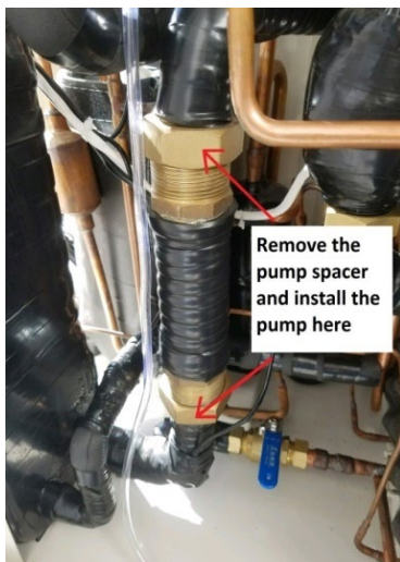
Removing the shipping spacer
