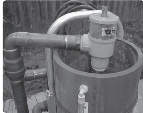
Figure 15: Cam Fittings for Flush Cart Hoses
