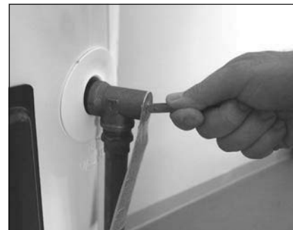
Figure 13 - T&P Relief Valve
