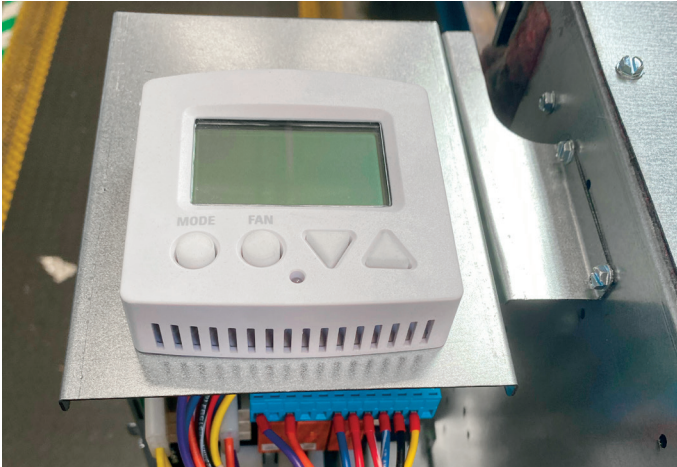
Figure 38: Thermostat unit-mount (Venture Wi-Fi Thermostat mounted on LHA)
