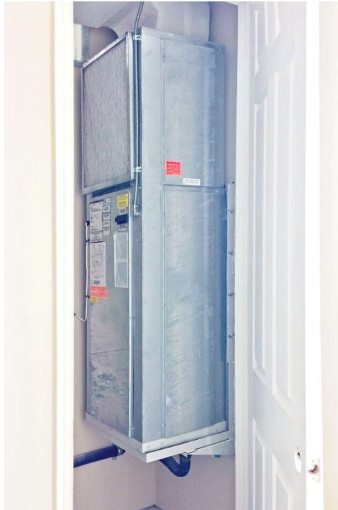
Figure 14- Sleeve with condensate drain line
