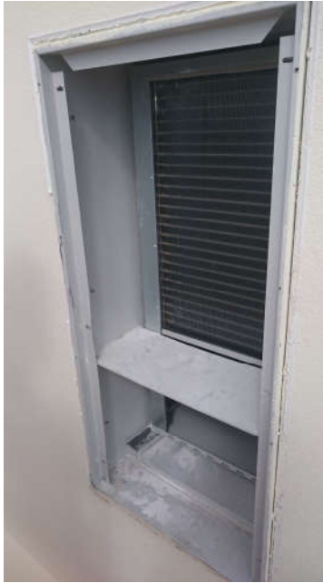
Figure 11 – Exterior Wall sleeve installation
