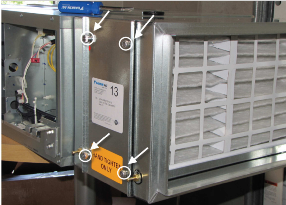
Figure 6: To utilize meter connections, remove the screws from the connection port and install the meter hose.
