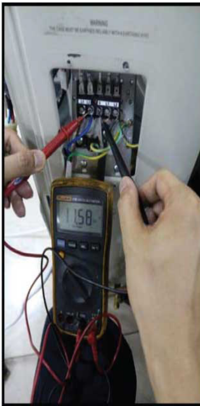
Fig. 17 —Test the DC Voltage
