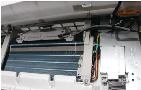
**Fig. 35 — Use ties to keep wiring aligned**
