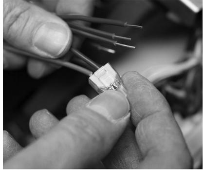
6. Using supplied wire nuts, attach wires from cell to wires from ballast. Matching blue to blue and red to red.
