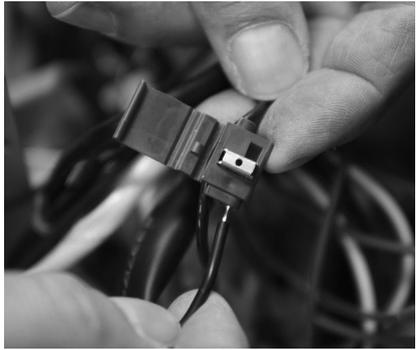
8. To use the wire tap splice terminal, first place around line voltage wires, then insert ballast wire, and press firmly. White to white and black to black. Tuck wiring from PTAC unit safely around the sheet metal and into the high voltage control panel.
