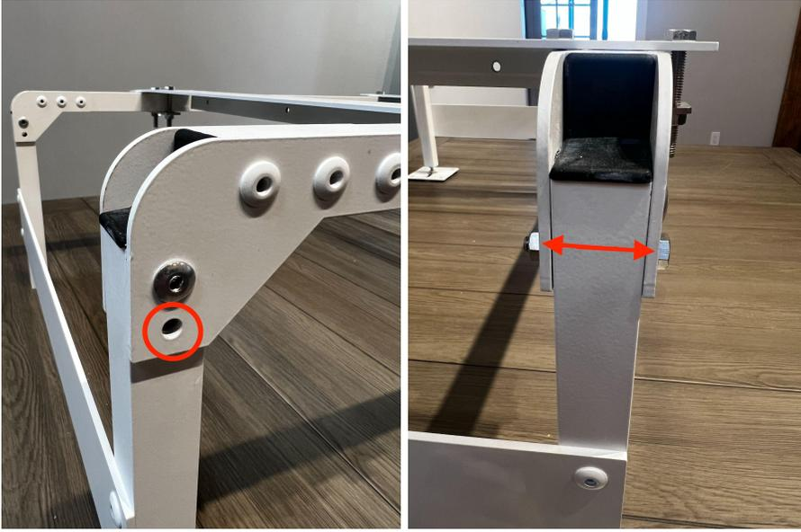
4. Adjust support channels to align with feet arrangement of heat pump and mount feet into channels using the provided 5/16" x 2.5" bolts, washers, nuts and vibration isolation pads
