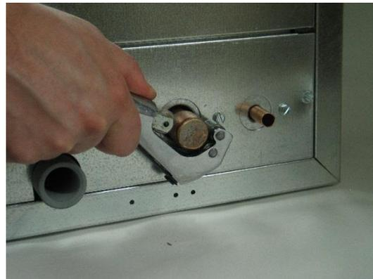
**Figure 22. Cut end of connection as shown.**
