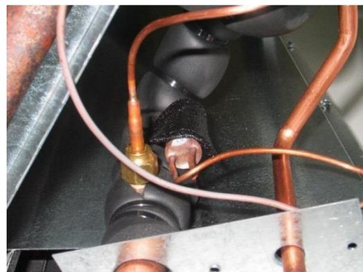
**Figure 30. Bulb Secure Clamp and Cork Tape**
