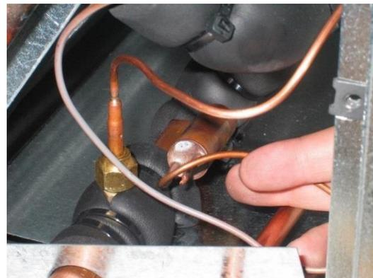
**Figure 29. Thermal Measuring Bulb Placed on Copper Tube.**
