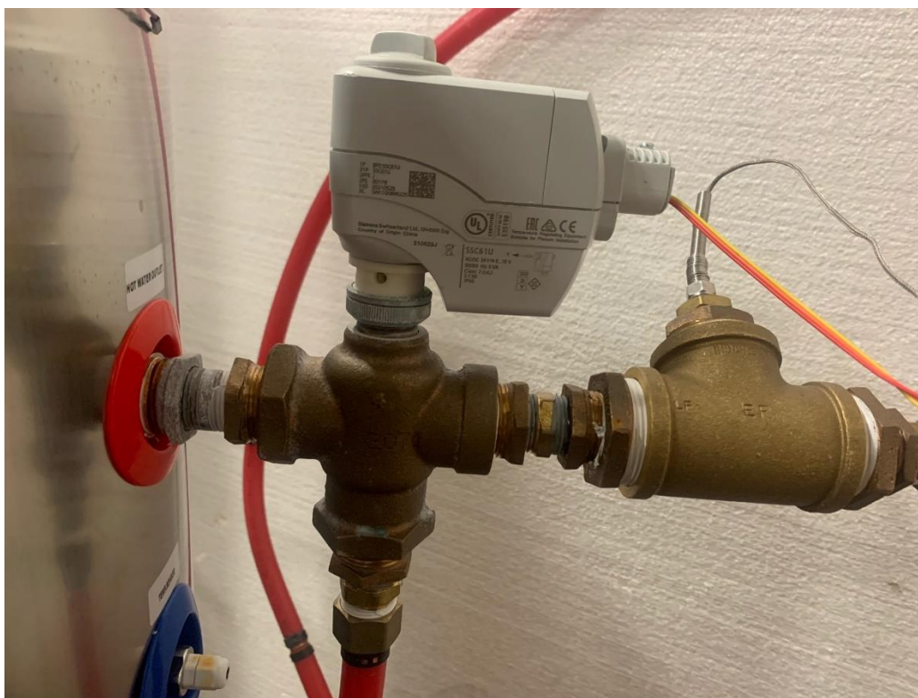
Above, valve supported by copper pipe on 2 sides
