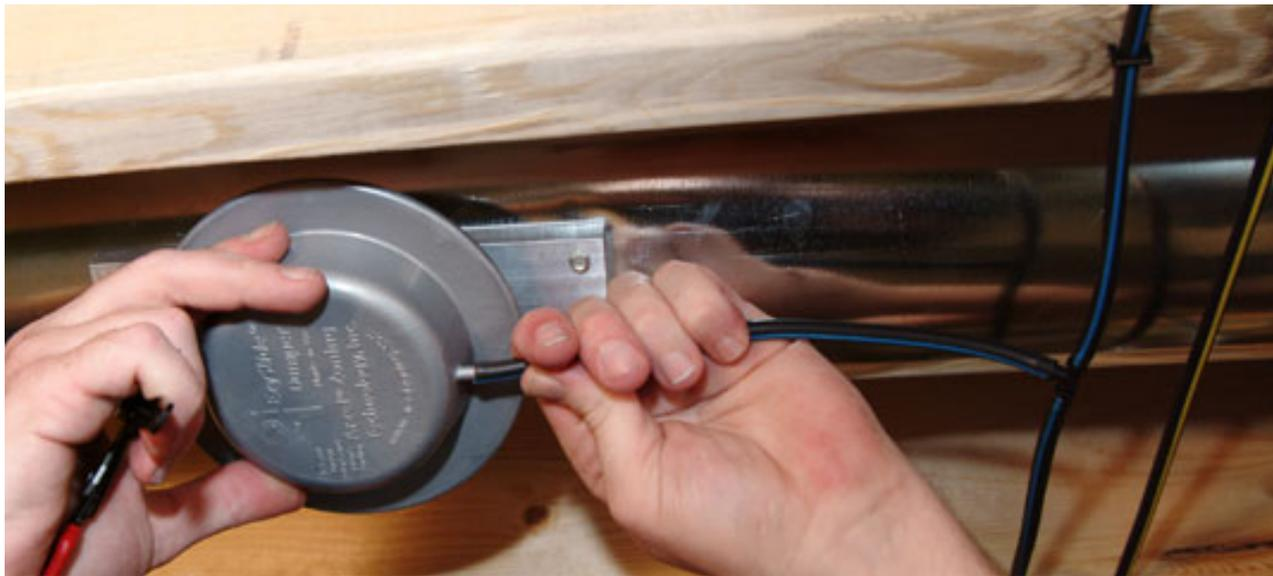
Cut a  $\frac{3}{4}$ " section out of the "Homerun Tube" for that zone and insert a tee to connect to damper
