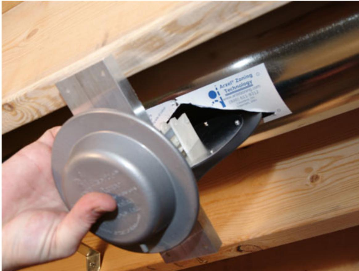
With the damper being held in the “Closed” position, insert with the blade at the wide end of the triangle
