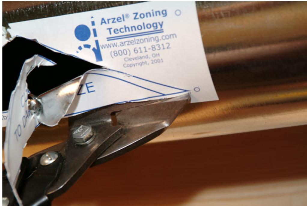
Drill a  $\frac{3}{4}$ " hole at each of the three corners and connect the holes with your snips
